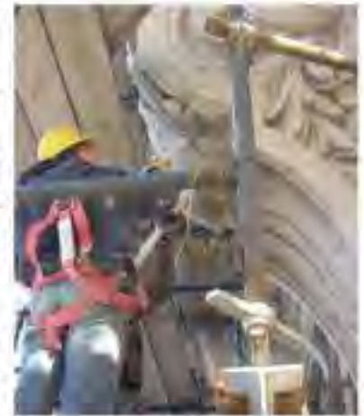
Grout being pumped into the terra cotta anchor assembly to engage and stabilize terra cotta units.
